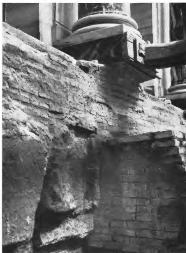
Fig. 192 — S. Marco. Third-period nave foundations; stylobate resting on Servian blocks (Photo: Soprintendenza ai monumenti).
